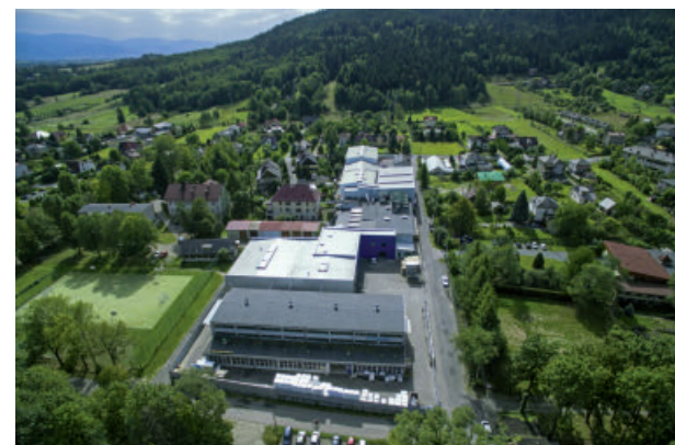
Buczkowice – production & warehouse
